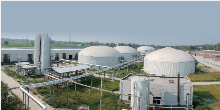
Processing capacity: manure and straw 1000 t/d
